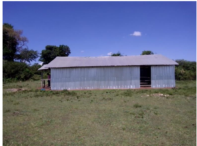
Ilabur Lighthouse Baptist Church – Masai, with no windows at the moment
